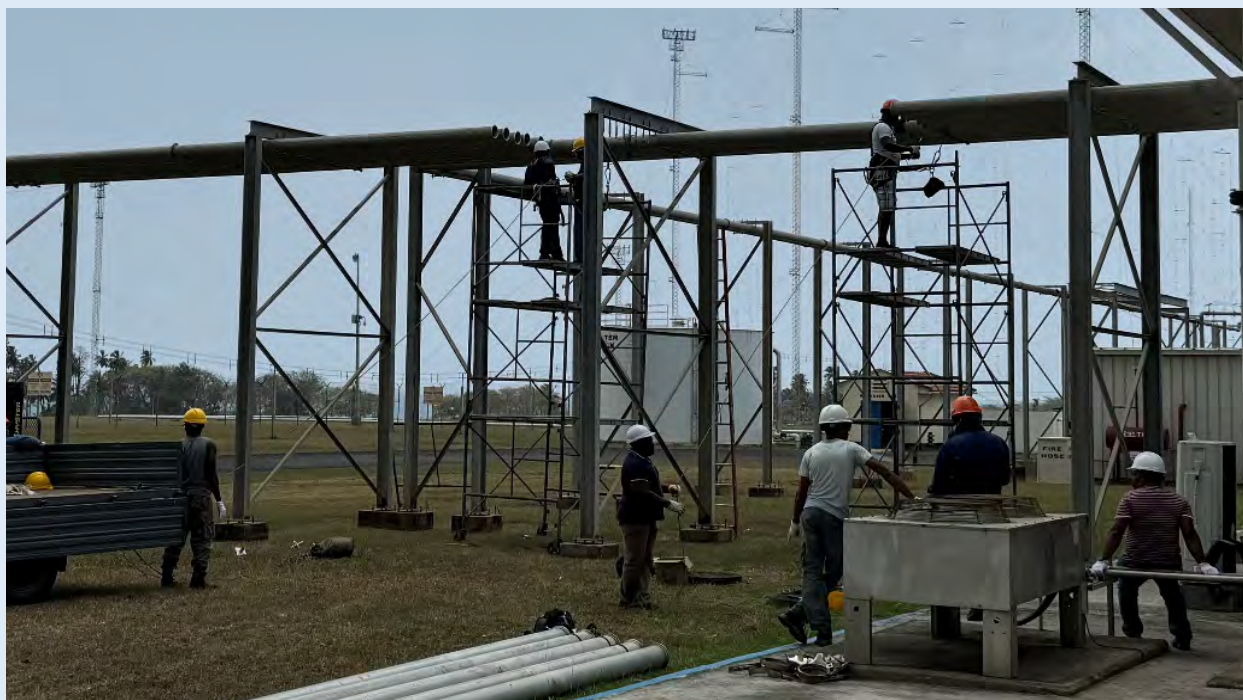
Work crew in Sao Tome dismantling transmitter cabling from USAGM shortwave radio towers and antenna systems (seen in background).
