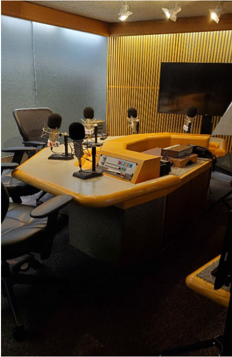
Figure 10 shows a typical on-air live studio with microphones for up to five speakers.
